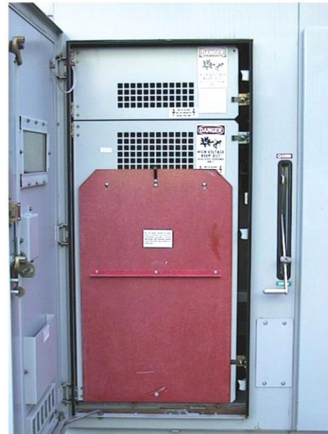
16K – Figure 2 Isolation Barrier in Storage Position
