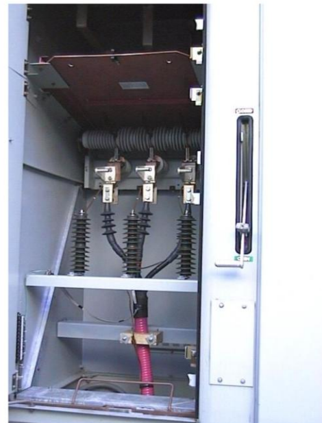
16K – Figure 4 Barrier Isolating Switch
