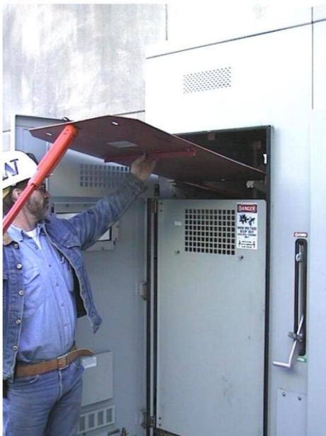
16K – Figure 3 Isolation Barrier Being Inserted
